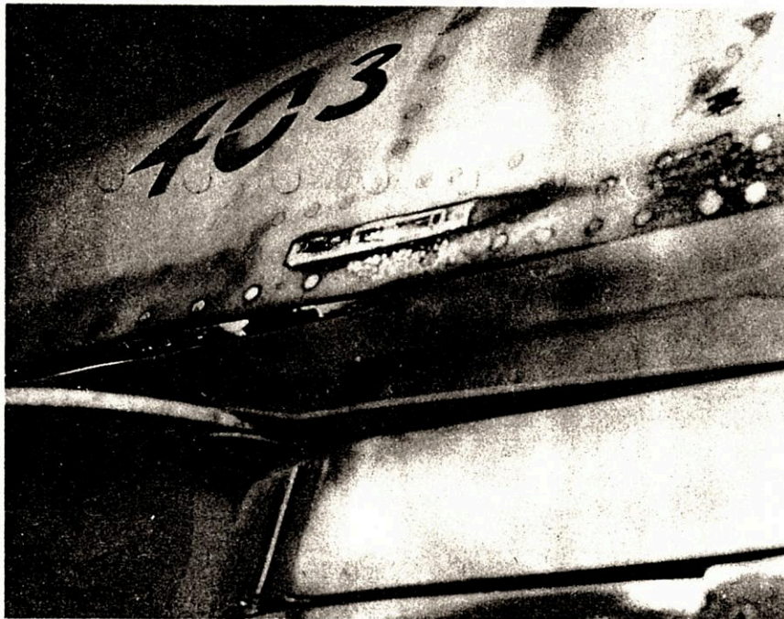
FIG. 39 - DAMAGED LATCH AND SEAM OF FORWARD STRUT FAIRING, EXTERNAL LEFT SIDE VIEW
