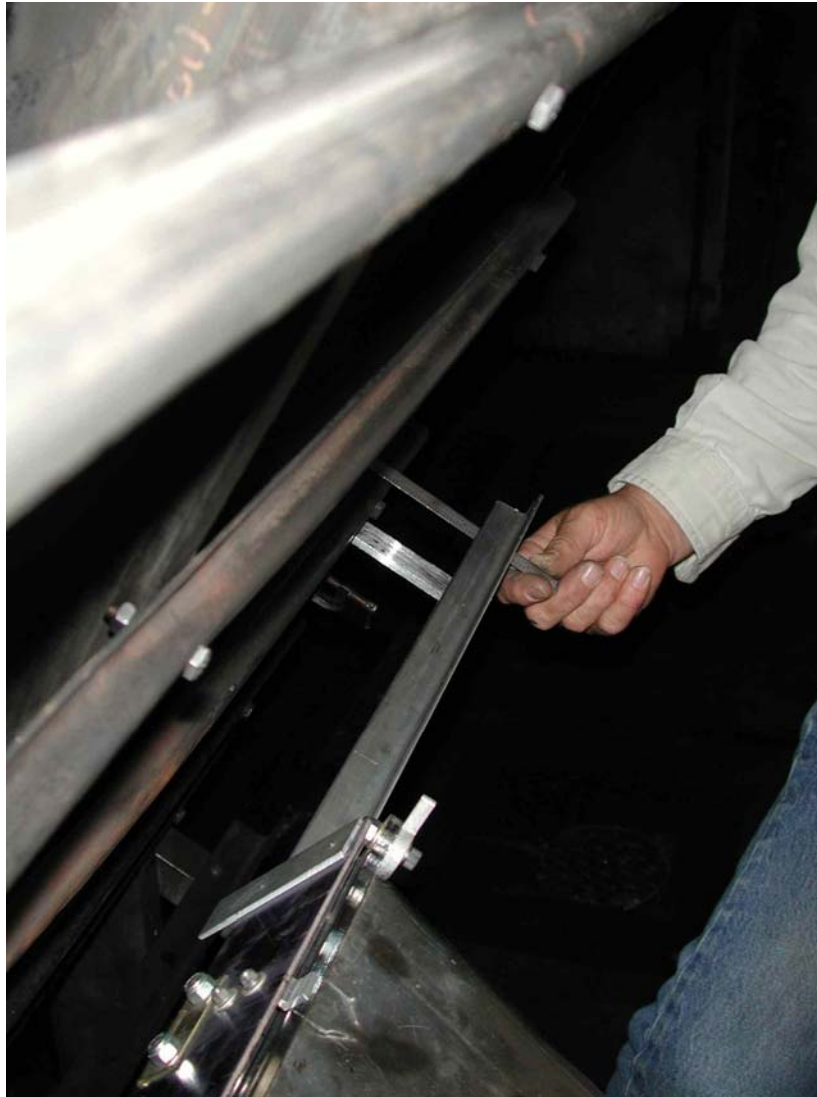
Figure 12. Measuring Distance to Outer Formers
