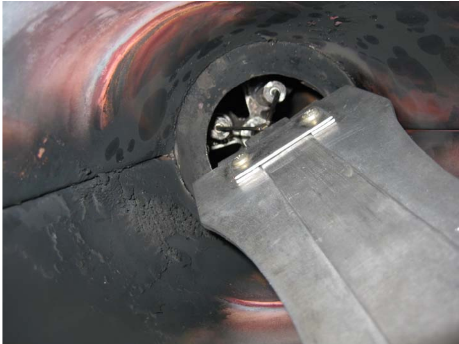
Figure 6. Checking Ignitor Depth
