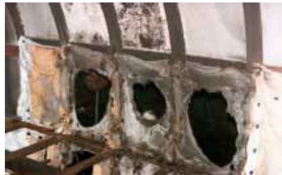
Burn Test with Ineffective Insulation
