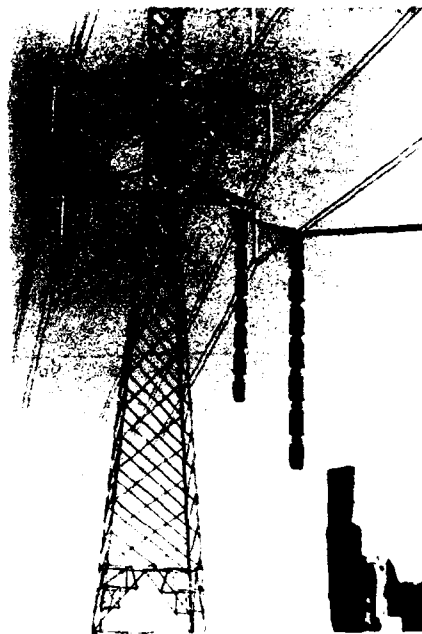
Fig. 14 Anti-torsional device for single layer armored OPGW
