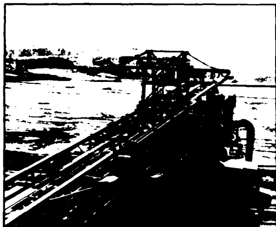
Fig. 2: Bridge from the digger to the conveyor road
