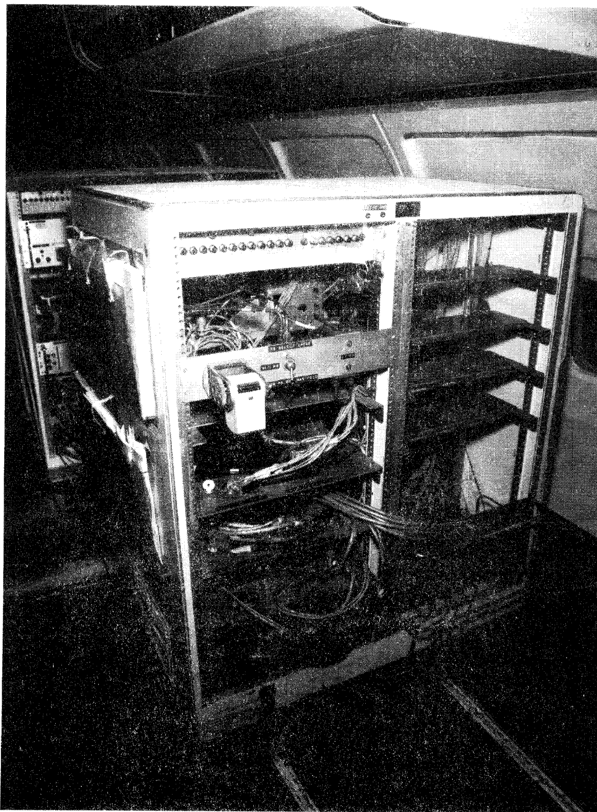
FIGURE 2.1.1-5 INSTRUMENT RACK, STATION 1386, LEFT SIDE
