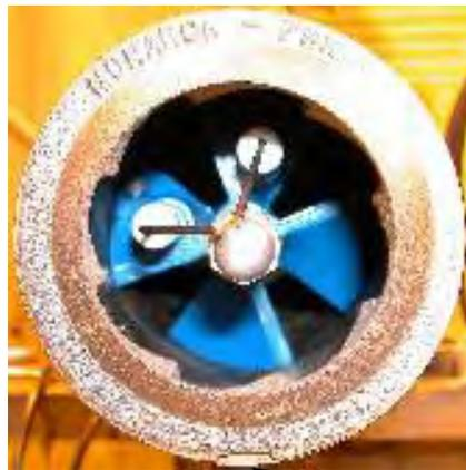
Turbulator Alignment Notch
