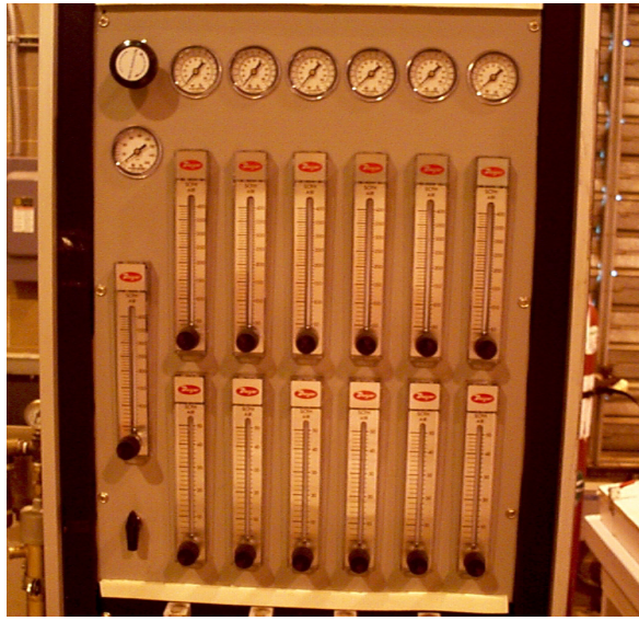
FIGURE 7. NEA DEPOSIT MANIFOLD CONTROL PANEL
