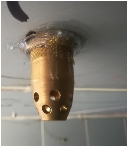
Nitrogen spray nozzle and nitrogen supply arrangement
