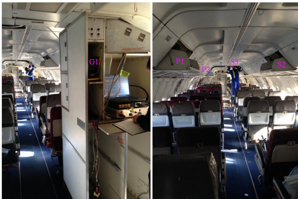
a) Computer and heater control in aft galley b) Heater installation in bins, seats, attic
