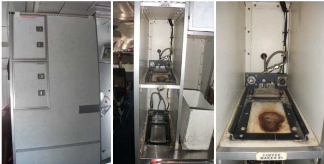
a) Aisle side of galley cabinet b) Coffee maker bays c) Heat damage on upper bay
