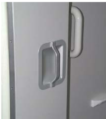
Figure 12. The embedding type handrail equipped on the toilet outer wall
