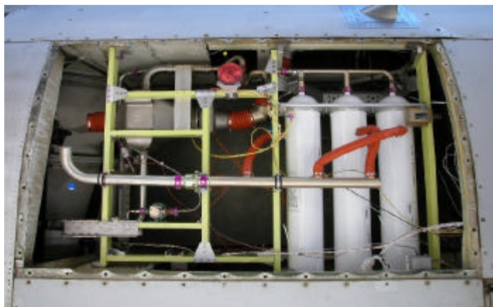
Figure 2. OBIGGS Installed in Boeing 747 SP Ground Test Article Pack Bay
