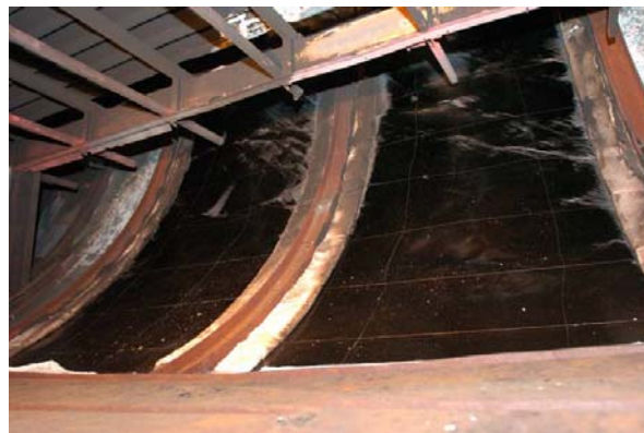
Figure 7. Burnthrough Resistance of Composite Fuselage Subjected to a Jet Fuel Fire for 5 Minutes
