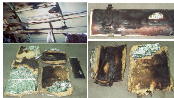
Figure 1. Hidden In-Flight Fire Incident Involving Thermal Acoustic Insulation
