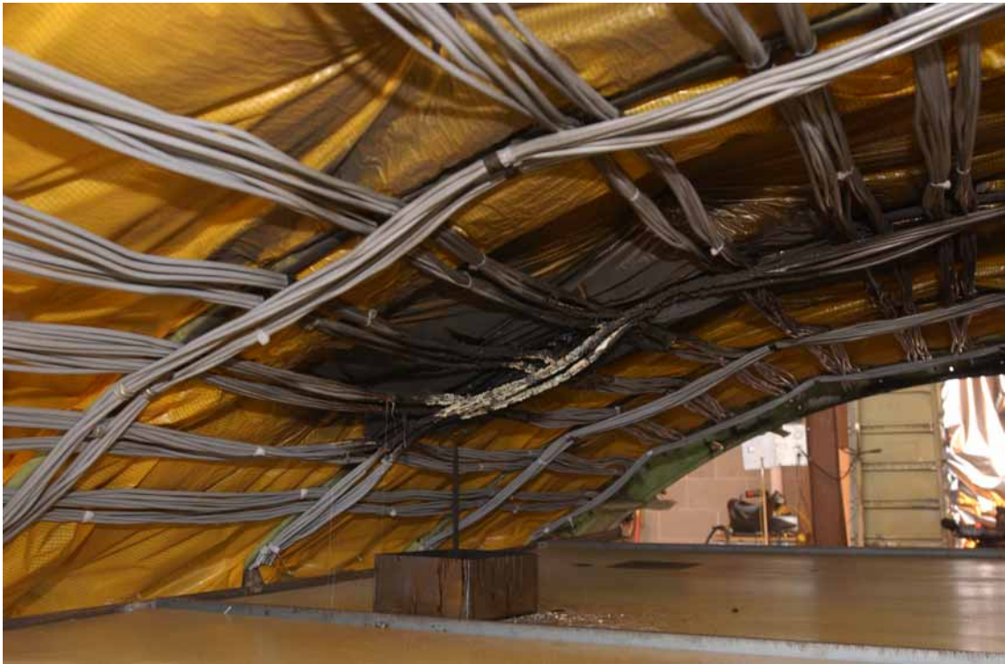
FIGURE 21. FLAMEOUT OF RISER CABLE (A)
