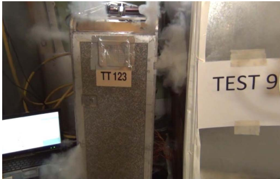
Figure 41. Thermal runaway event
