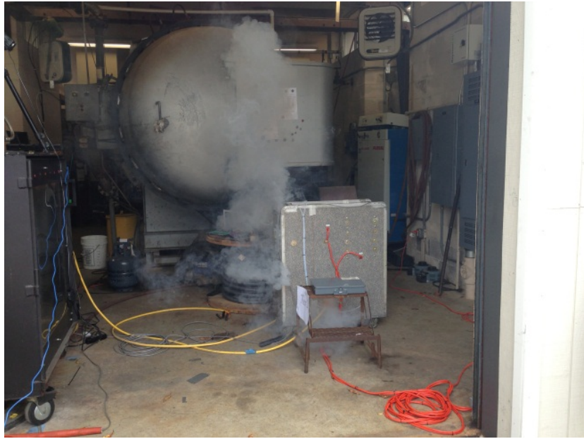
Figure 16. Thermal runaway event within the cart
