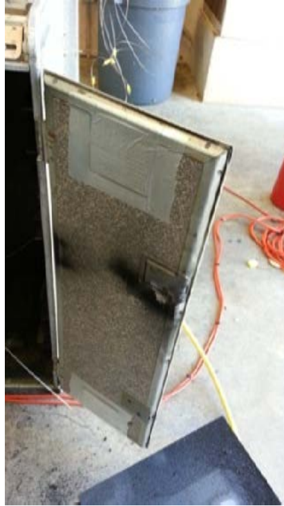
Figure 35. Soot marks from the fire
