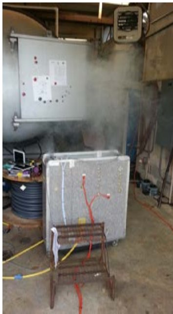
Figure 20. Thermal runaway event within the cart
