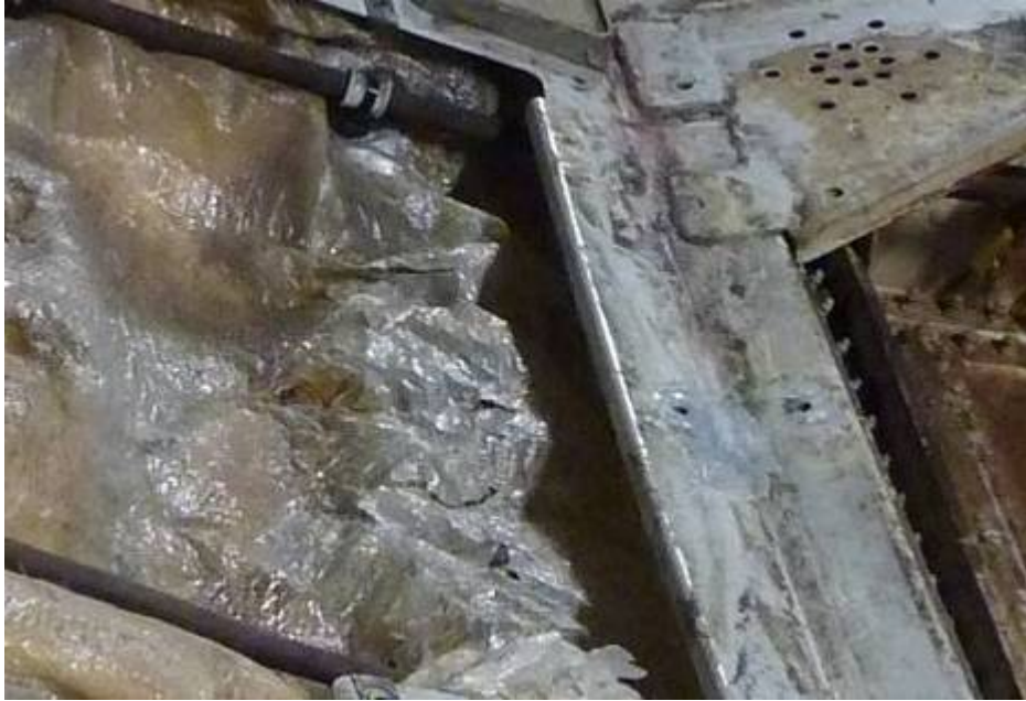
Figure 23. Degraded TAI in 'Wet' Area in Fuselage Keel
