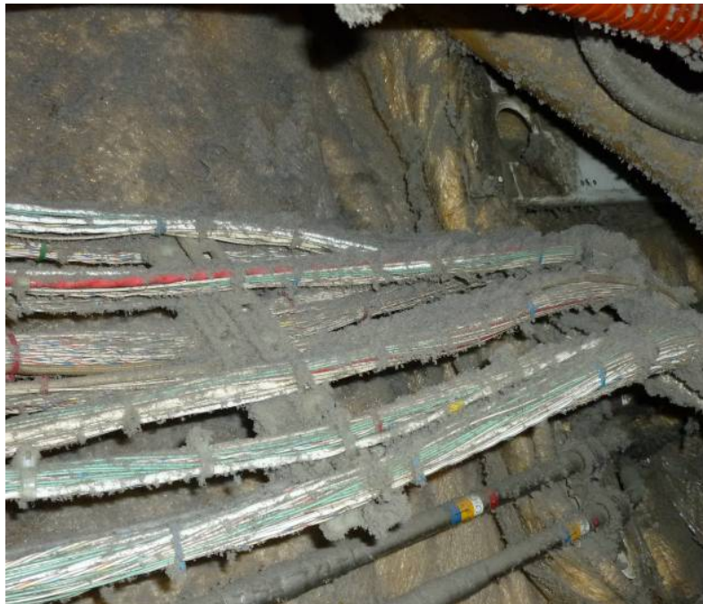
Figure 37. Significant Accumulations of Dust and Lint on TAI and EWIS Near to Cabin Air Recirculation Inlet in the Under-Floor Cheek Area
