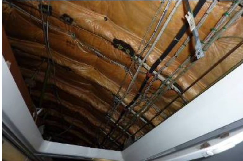
Figure 11. Clean TAI and EWIS Above Cabin Ceiling
