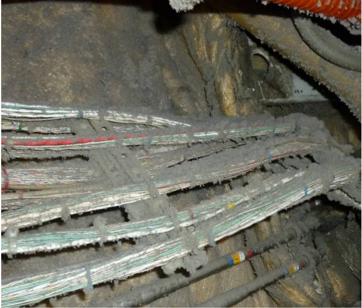
Figure 16. Significant accumulations of Dust and Lint on TAI and EWIS Near to Cabin Air Recirculation Inlet in the Under-Floor Cheek Area
