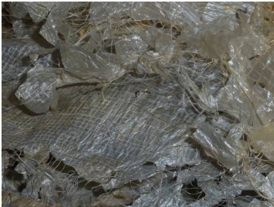
Figure 24. Exposed Reinforcing Scrim on Degraded TAI
