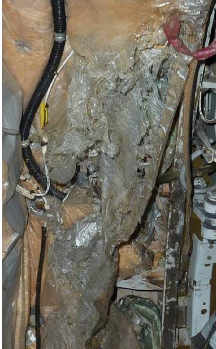
Figure 22. Degraded TAI in 'Wet' Area Near Passenger Door Surround
