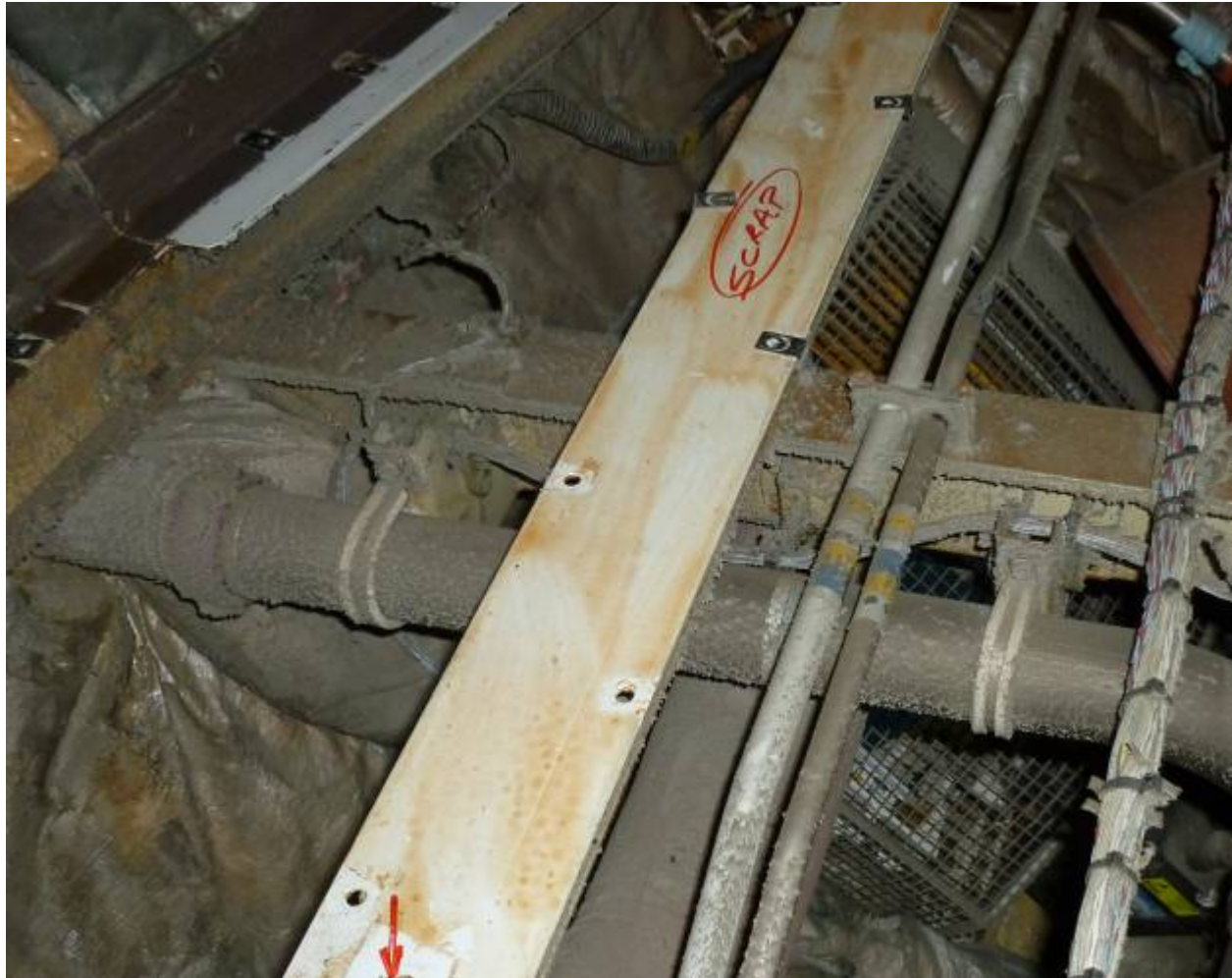
Figure 15. Significant Accumulations of Dust and Lint on TAI, EWIS, and Structure Near to Cabin Air Outflow Valve (Outflow valve is located behind mesh guard)
