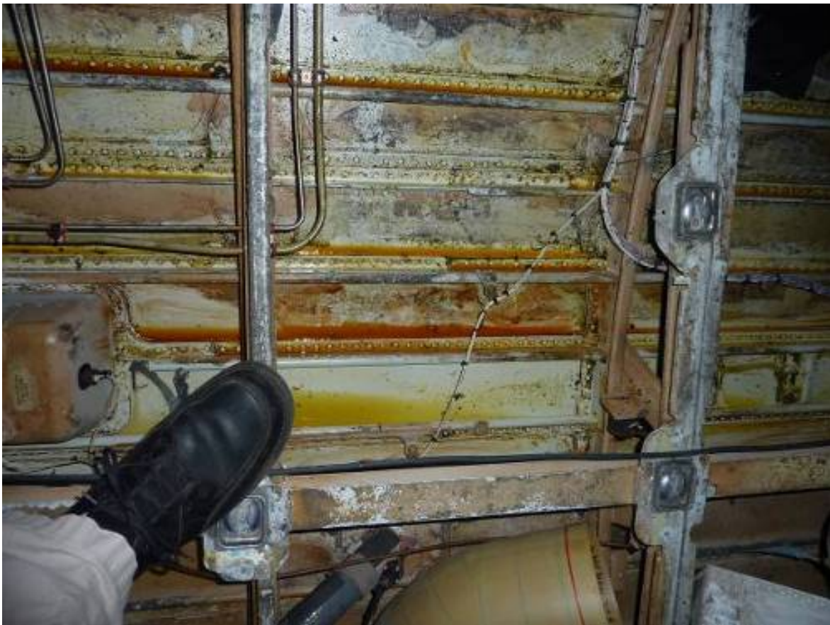
Figure 21. Pools of CIC Dissolved by Hydraulic Fluid in Keel Structure
