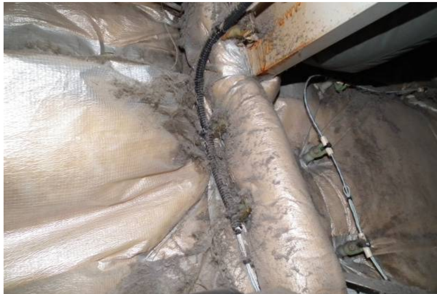
Figure 14. Dust and Lint Accumulation Below Cabin Floor
