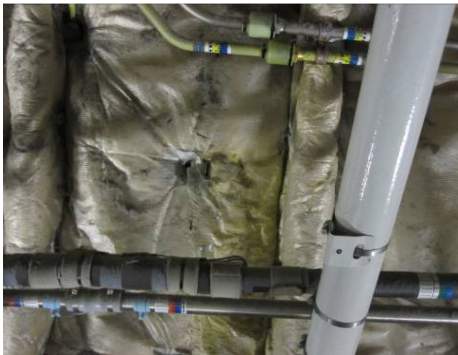
Figure 9. TAI Contaminated with Hydraulic Fluid
