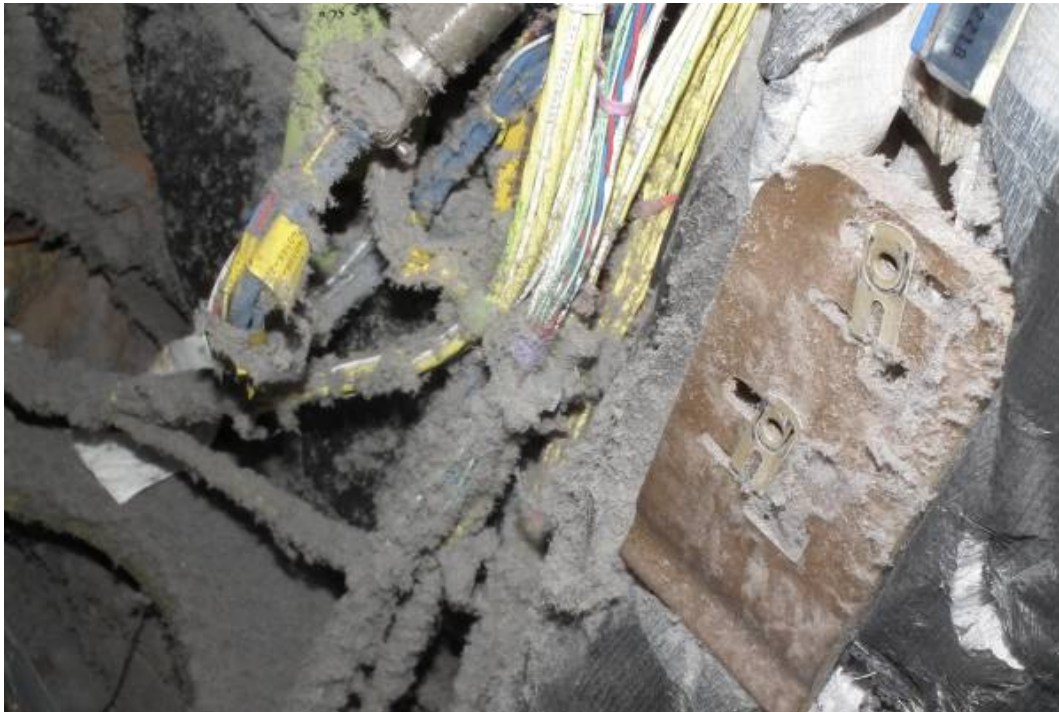
Figure 32. Dust and Lint Contaminated EWIS and TAI
