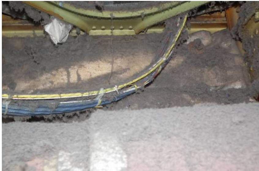
Figure 13. Dust and Lint Accumulation Below Cabin Floor
