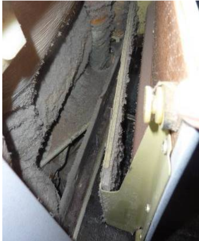
Figure 10. Dust and Lint Deposits Behind Dado Panel
