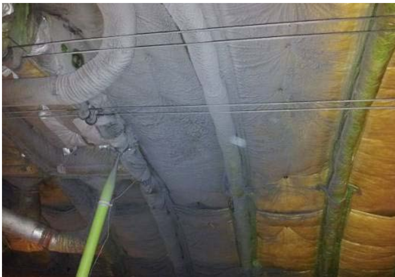
Figure 12. Dust and Lint Above Cabin Ceiling Ejected From Air Recirculation Outlet
