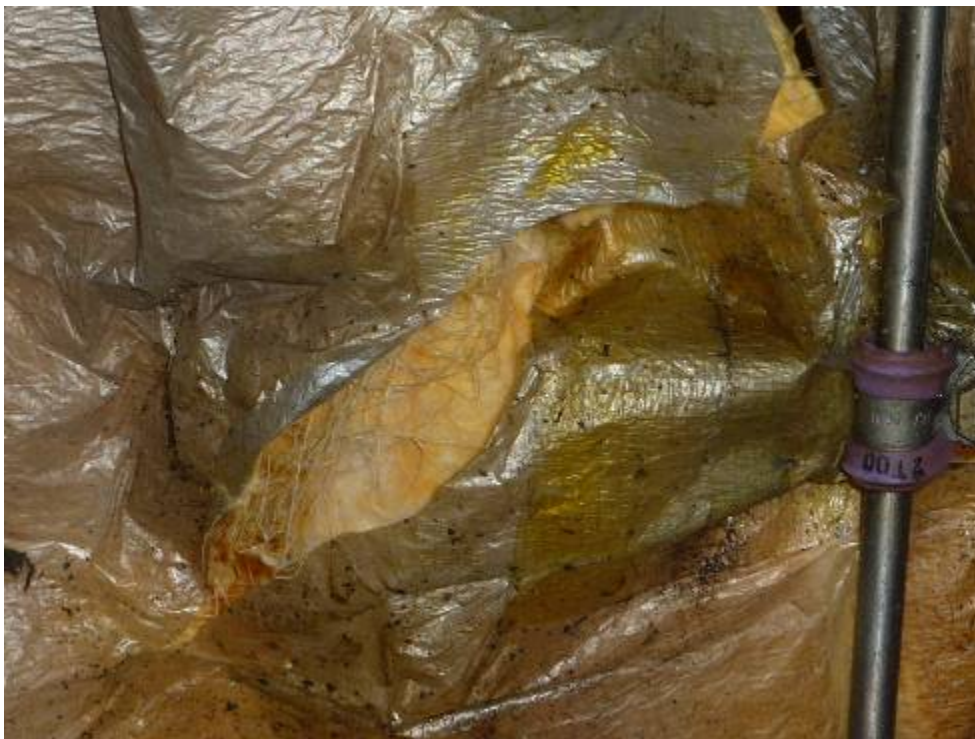
Figure 18. Hydraulic Fluid Leakage and Damaged TAI
