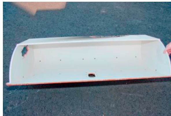
Figure A-9. Inserts Inside a Stowbin for Attaching Trim
