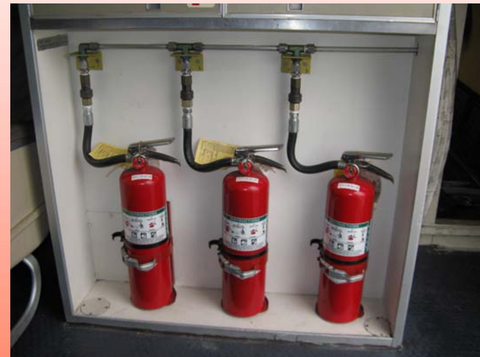
Halon bottles in front of barrier
