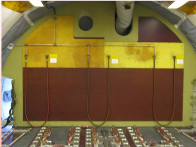
Halon hoses in Class E compartment
