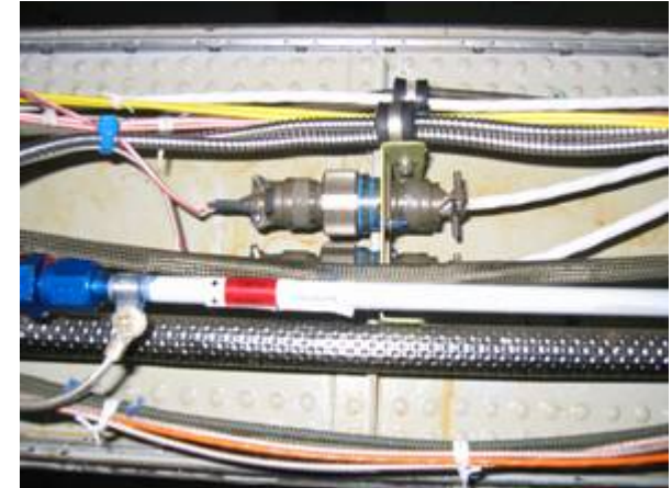
Temperature Wires Connectors
