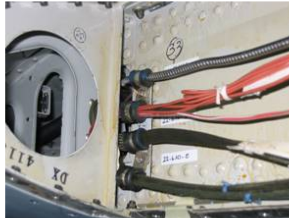
Fuel Venting Box Probe
