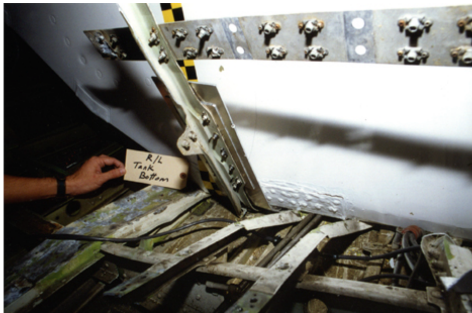
FIGURE A-30. FUEL TANK—BOTTOM, LEFT REAR
