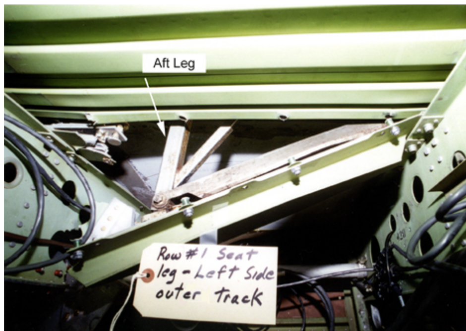
FIGURE 26. DISPLACEMENT OF OUTER SEAT TRACK INTO CARGO AREA
