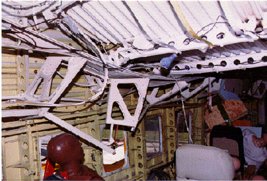
FIGURE 33. CEILING DEFORMATION POSTTEST PILOT SIDE
