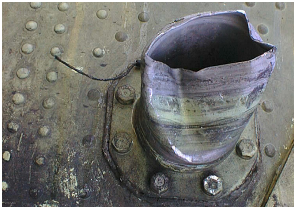
FIGURE 16. CELL 4 INTERCONNECT FITTING DAMAGE
